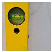
Level the joint in the whole vertical direction to ensure a correct arrangement of the panels.
