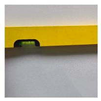
Level the joint in the whole horizontal direction to ensure a correct arrangement of the panels.
