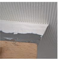
Spread the adhesive onto the wall with a notched trowel (i.e. 2.3 x 2 mm notches at 5 mm on center, check the suppliers datasheet).
