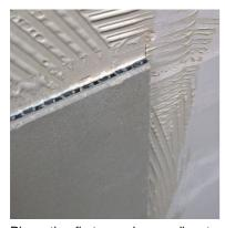
Place the first panel according to the marked cross joints by slightly twisting it into the adhesive and thereby ensure a good overall contact.
