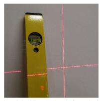
Level the joints in the whole vertical and horizontal direction to ensure a correct arrangement oft he panels.
