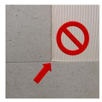
Avoid higher amounts of adhesive material in the panel joint area to prevent a penetration of adhesive through the joints. Also avoid spreading adhesive tot he panels surface while completing the wall arrangement. Adhesive needs tob e removed before curing by using a clean cloth and rubbing alcohol.
