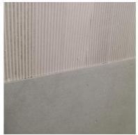
Place the first panel according tot he marked cross joints by slightly twisting into the adhesive and thereby ensure a good overall contact. Based in correct position, press the panel firmly into the adhesive.
