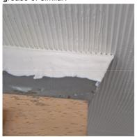
Spread the adhesive onto the wall with a notched trowel (i.e. 2.3 x 2 mm notches at 5 mm on center, check the suppliers datasheet).
